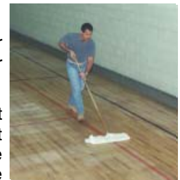
Tacking floor with cotton towels and push broom.
