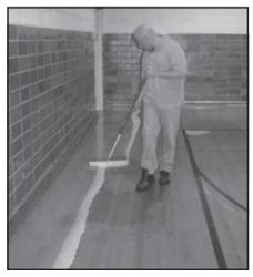
4. Rinse floor with plain water and a well 5. Tack the floor with plain water and 6. Apply finish. For Court Shield waterborne products, wait 1 hour after tacking floor. For Poli-Mirro 450, wait overnight before applying.
