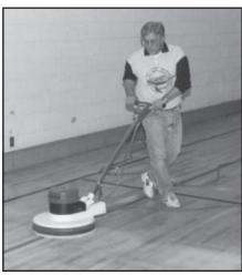
1. After dust mopping, begin the process 2. Scrub the solution with a 120 grit 3. Immediately pick up solution with a screen under a 175 rpm floor machine. Overlap each area slightly. Flip screen after 250 sq. ft.
