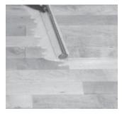
begin applying by pushing the excess finish toward the opposite side of the floor (snowplowing). Continue pouring and applying product across the floor. Take care not to allow excess product to flow off the applicator on
