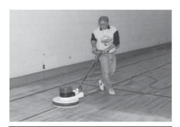
**TIP:** If possible, shut off the ventilation system in the gym during application of finish to minimize air borne dust settling into the wet finish. Turn back on when the finish begins to set to aid drying.
