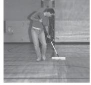
product is on the floor, collect it near the exit point and soak up with towels or rags. Do not attempt to feather this excess product onto the floor.
