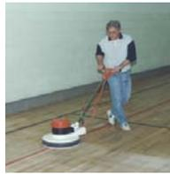
One screen is required for every 500 square feet (250 square feet/side). Screen floor two times in opposite directions for uniform results.
