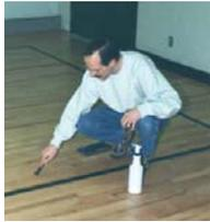
**Step 2:** Divide floor into smaller sections so Hi-Trac solution does not dry out before being picked up. 250 square feet sections are suggested.
