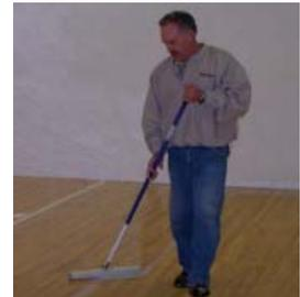
Do not to allow excess product to flow beyond the opposite end of the applicator at the end of each run. If this happens, gently squeeze out excess product from the applicator, then gently feather out the excess material on floor.
