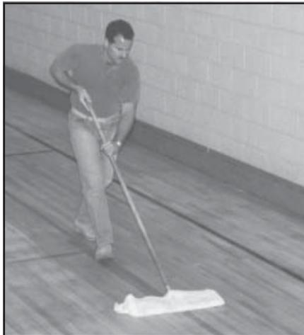
5. Tack the floor with plain water and large white towels to remove remaining residues. Repeat process until floor is clean. To test if floor is clean, wipe floor after it has dried with bare hand. If residue is found, repeat.
