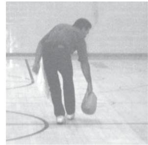
**Step 2.** Pre-wet the applicator in the line of finish then begin applying by pushing the excess finish toward the opposite side of the floor (snowplowing). Continue pouring and applying product across the floor. Take care not to allow excess product to flow off the opposite end of the applicator on
