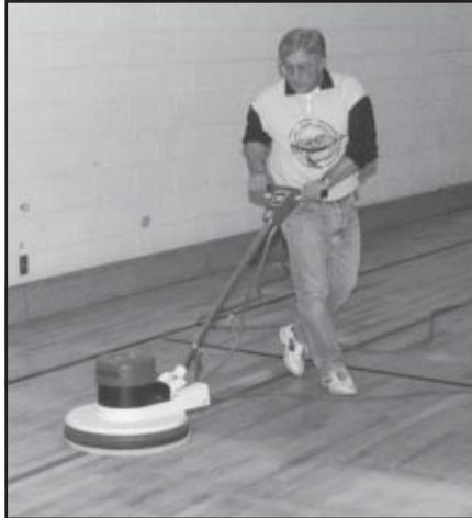
2. Scrub the solution with a 120 grit screen under a 175 rpm floor machine. Overlap each area slightly. Flip screen after 250 sq. ft.
