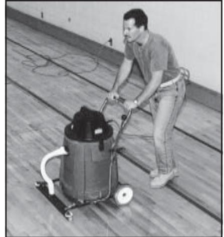
3. Immediately pick up solution with a wet/dry vac. Do not allow solution to dry on floor. Continue working 20'x20' areas. **Remember:** Change screens every 500 sq. ft.
