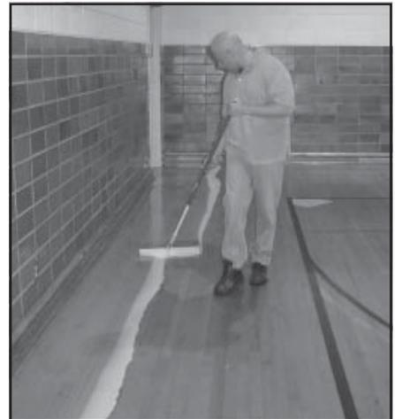
6. Apply finish. For Court Shield waterborne products, wait 1 hour after tacking floor. For Poli-Mirro 450, wait overnight before applying.
