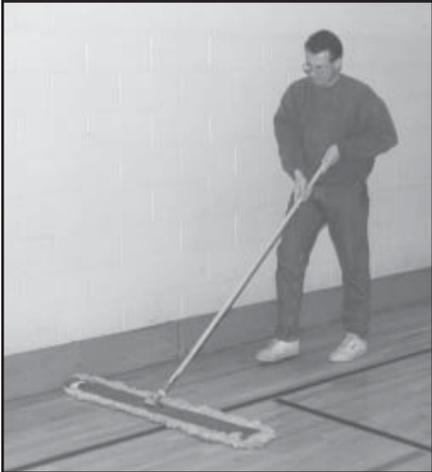
1. After dust mopping, begin the process by applying a solution of Hi-Trac at 4-6 oz./gal. with a mop. Work a 20'x20' section.
