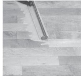
turns at the end of each run. If this happens, gently squeeze out excess material from the applicator, then gently feather out the excess material on the floor.
