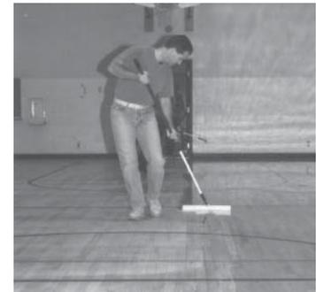
**Step 4:** Allow the floor to dry 3-6 hours depending on air flow and humidity. Reapply a second coat as recommended.
